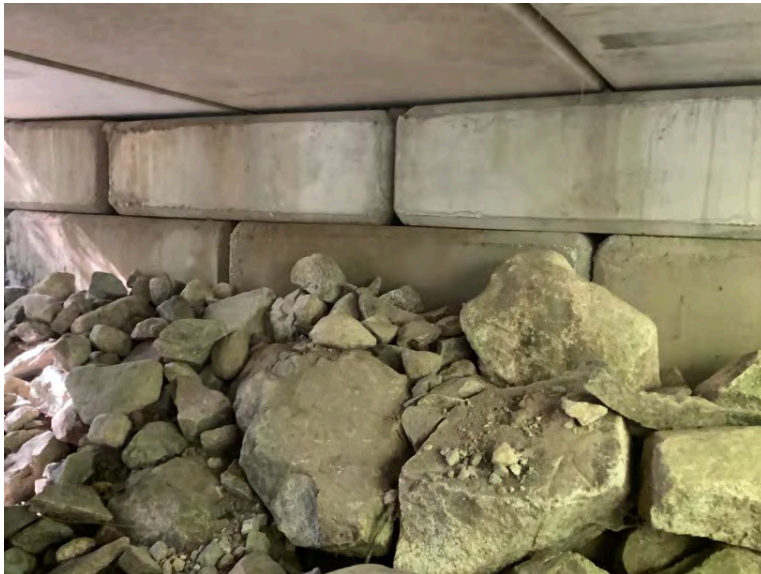
Right Bank Abutment when facing downstream
