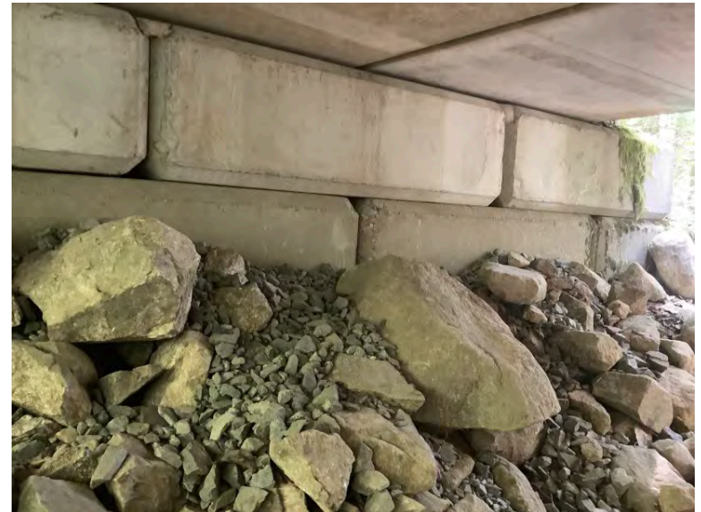
Left Bank Abutment when facing downstream
